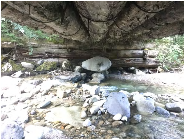
Left Bank Abutment when facing downstream
