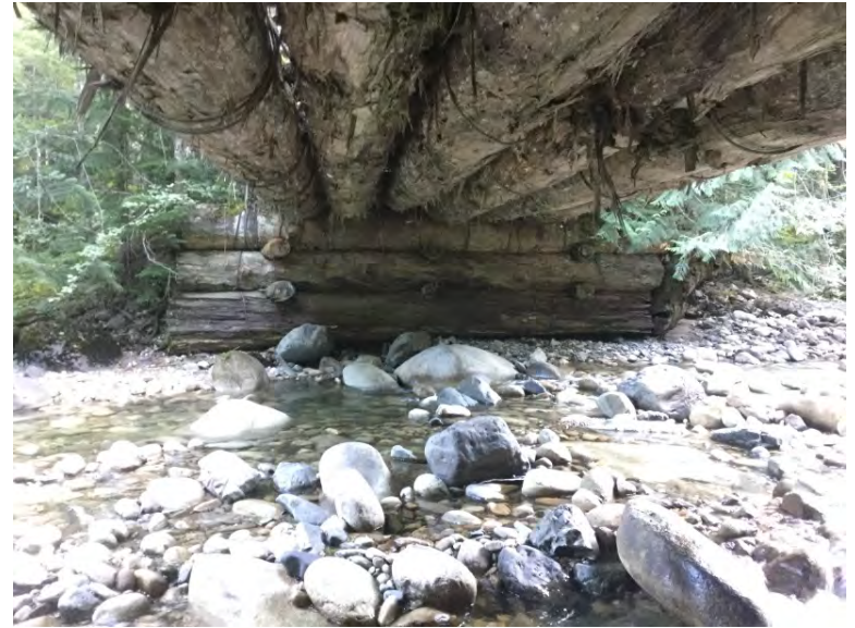
Right Bank Abutment when facing downstream
