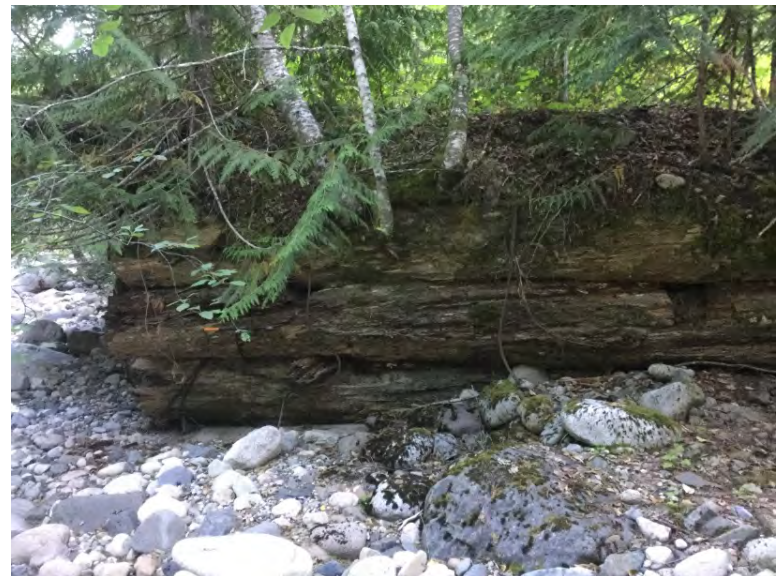
Upstream right bank wingwall condition
